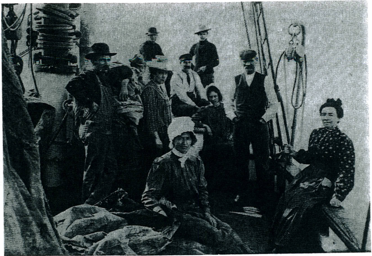
14. BOAT WITH TWO-YEAR SUPPLY OF OIL FOR CAPE MEARES LIGHT HOUSE AND SUPPLY OF GENERAL MERCHANDISE FOR THE PHELPS' STORE
