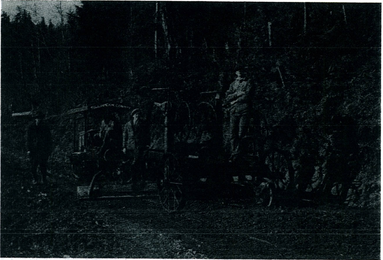
28. CONSTRUCTION OF ROAD TO OCEANSIDE
