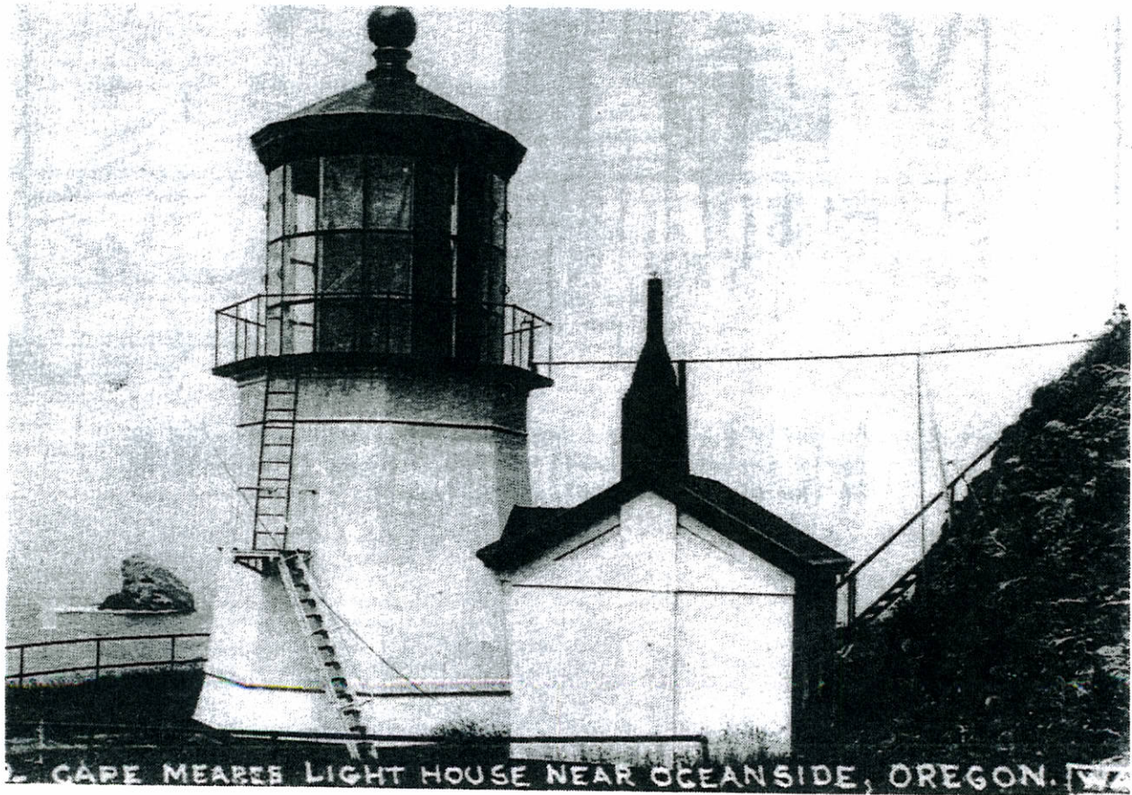
2. CAPE MEARES LIGHT HOUSE, CONSTRUCTED 1890-93
