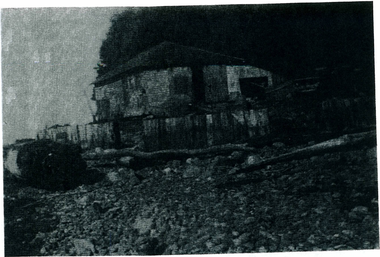
18. STORM DAMAGE, HAPPY CAMP
